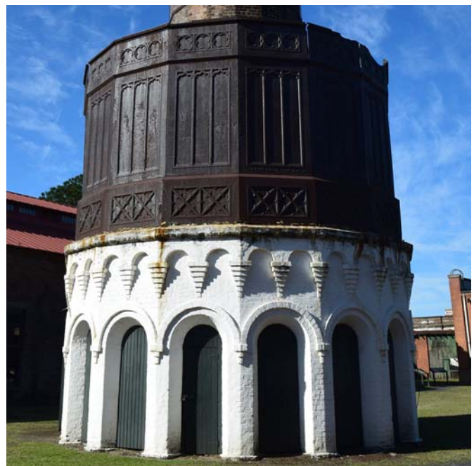
The towering smoke stack incorporates a water tank along with changing rooms and lavatories for shop roundhouse and shop employees.
